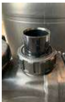
RACCORDEMENT POMPE Ø50
